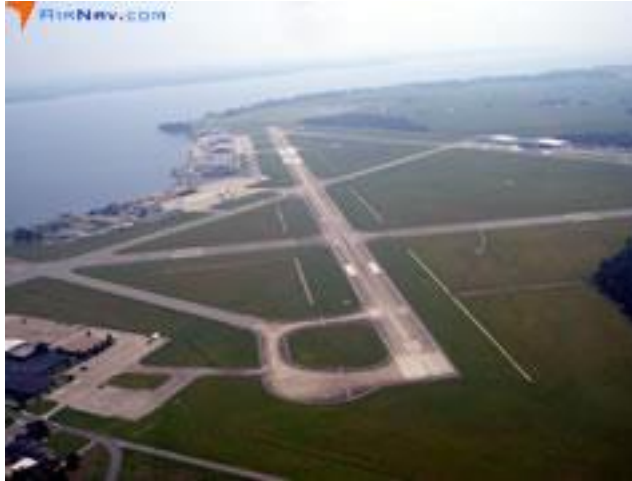
Coast Guard Station at Elizabeth City, NC
